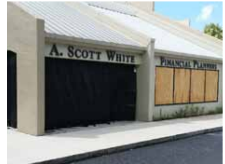
Before Irma, our office is secured.
